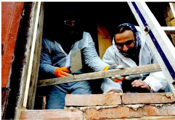
Fig. 3. Restoration of brickwork
