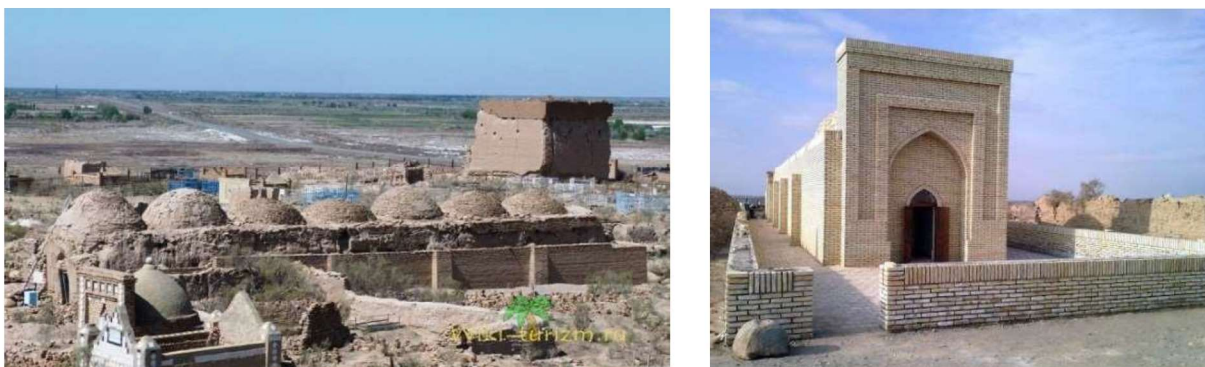
Figure 3. The mausoleum of Shamun Nabi: before and after repairing
