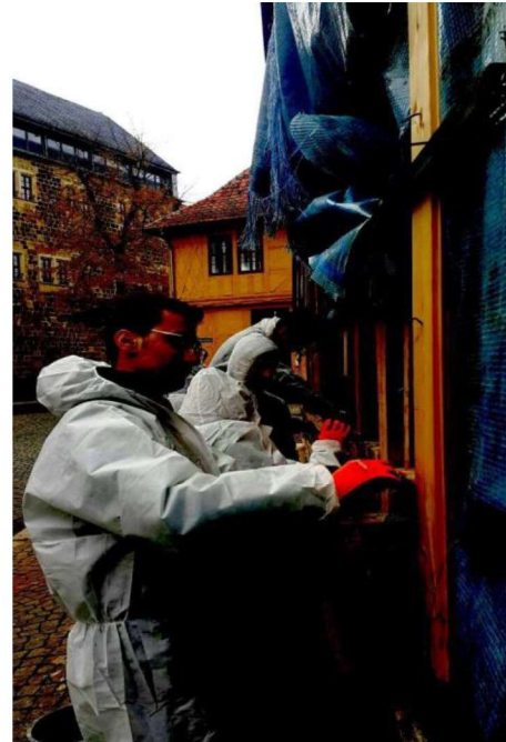
Fig. 2. Surface cleaning of a wooden column and treatment with a special solution
