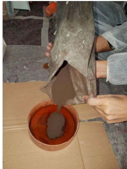
Fig. 4. Preparation of a special injection during restoration work
