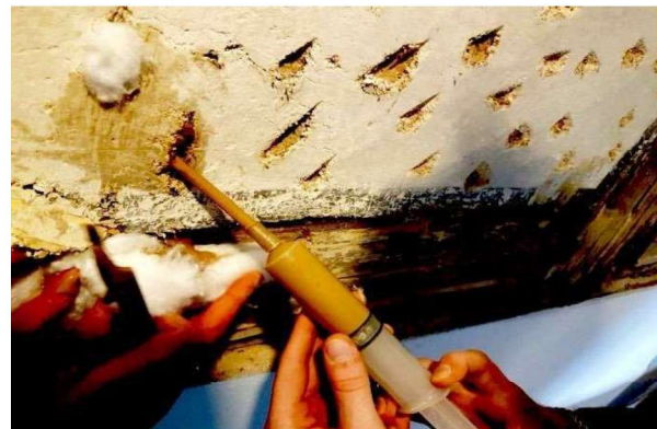
Fig. 5. Restoration work of a wooden frame and injection with a special solution
