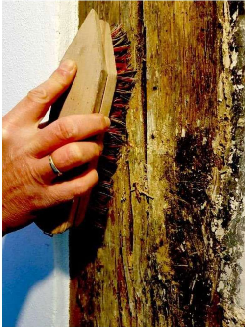
Fig. 2. Surface cleaning of a wooden column and treatment with a special solution
