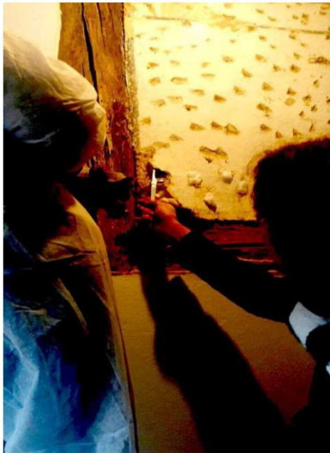
Fig. 6. Injection of a special solution into the filling attachment
