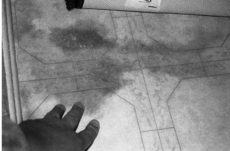
FIGURE 12.19 Linoleum discoloration due to moisture migration through a crack in the slab-on-grade foundation. The moisture accumulated beneath the linoleum at the location of the slab crack and caused the darkening of the linoleum as shown in the photograph.
