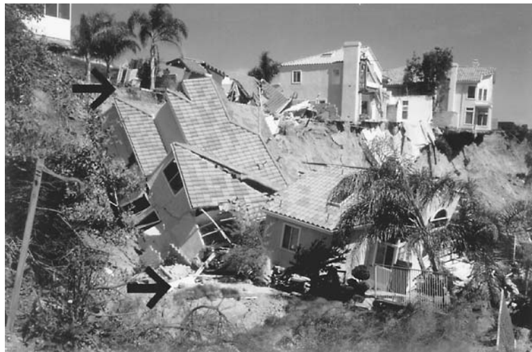
FIGURE 10.34 Laguna Niguel landslide: head of the landslide. (Note: The vertical distance between the two arrows is the distance that the landslide dropped downward.)
