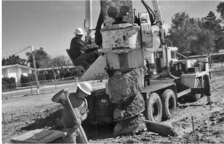
FIGURE 16.11 Close-up of auger being extracted from the ground with soil lodged within its grooves.
