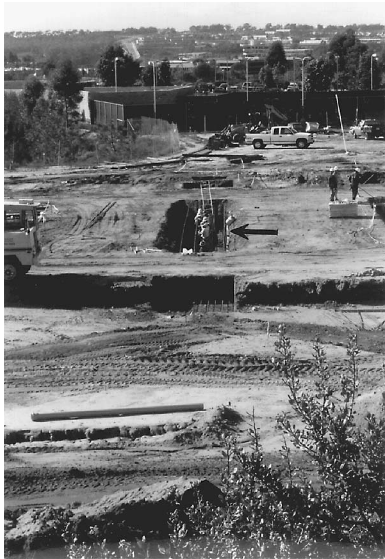
FIGURE 16.3 Installation of steel reinforcement in footings. The arrow points to the workers in the footing excavation in the process of installing the steel reinforcement.
