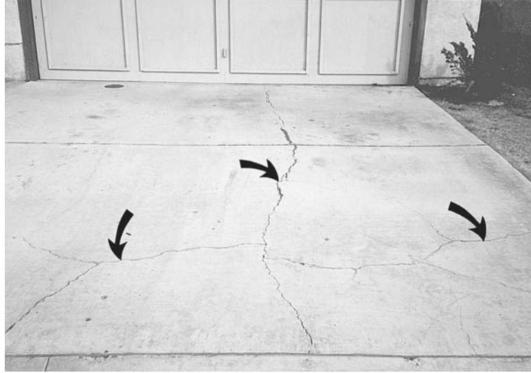
FIGURE 9.31 Driveway cracking due to expansive soil.
