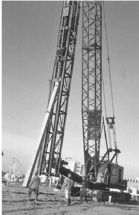
FIGURE 16.22 Pile driving equipment. A prestressed concrete pile is in the process of being hoisted into position.
