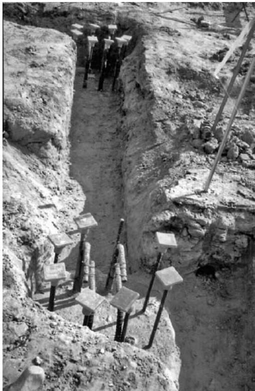
FIGURE 16.14 Excavation for the grade beam that will span between the two piers.
