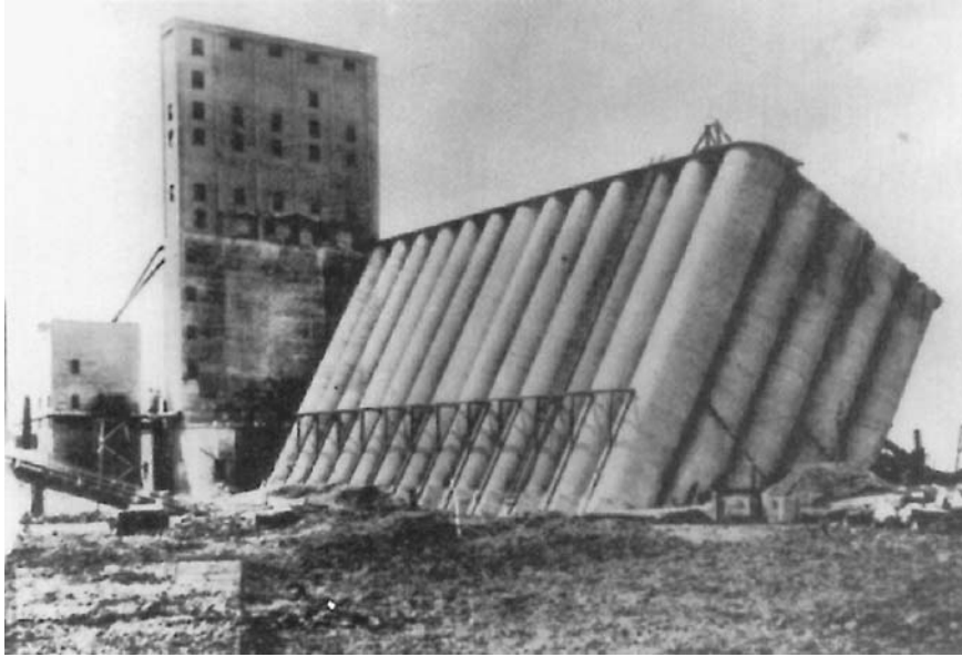
FIGURE 6.4 Transcona grain elevator failure.
