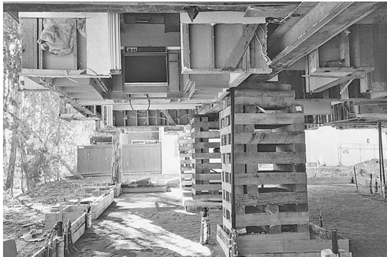
FIGURE 16.40 Construction of the mat foundation.
