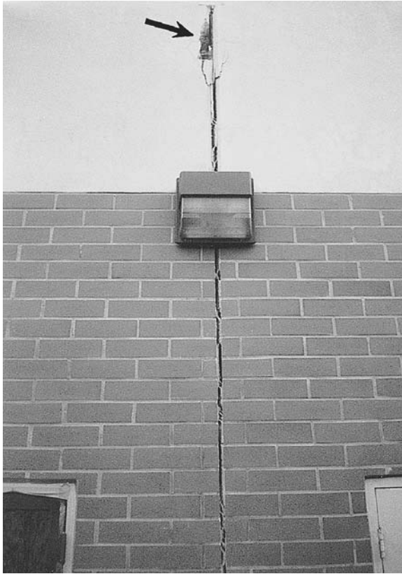
FIGURE 10.3 Joint separation between wall panels.
