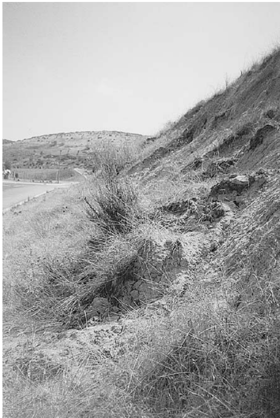
FIGURE 10.12 Surficial failure, cut slope for road.
