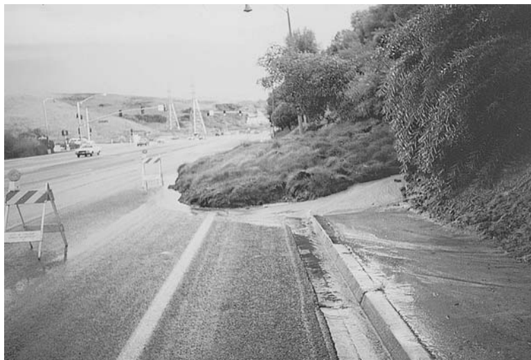
FIGURE 10.14 Partial mobilization of a surficial failure.
