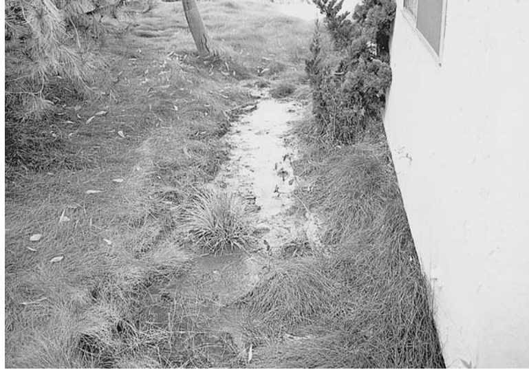
FIGURE 12.21 Poor surface drainage at a condominium complex.
