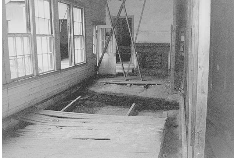
FIGURE 12.9 Drainage beneath parlor.
