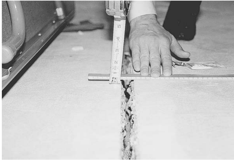
FIGURE 10.2 Damage due to lateral movement.
