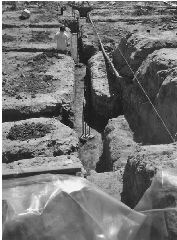
FIGURE 16.28 The excavation for the grade beams is complete and the top of the prestressed piles are trimmed so that they are relatively flush.
