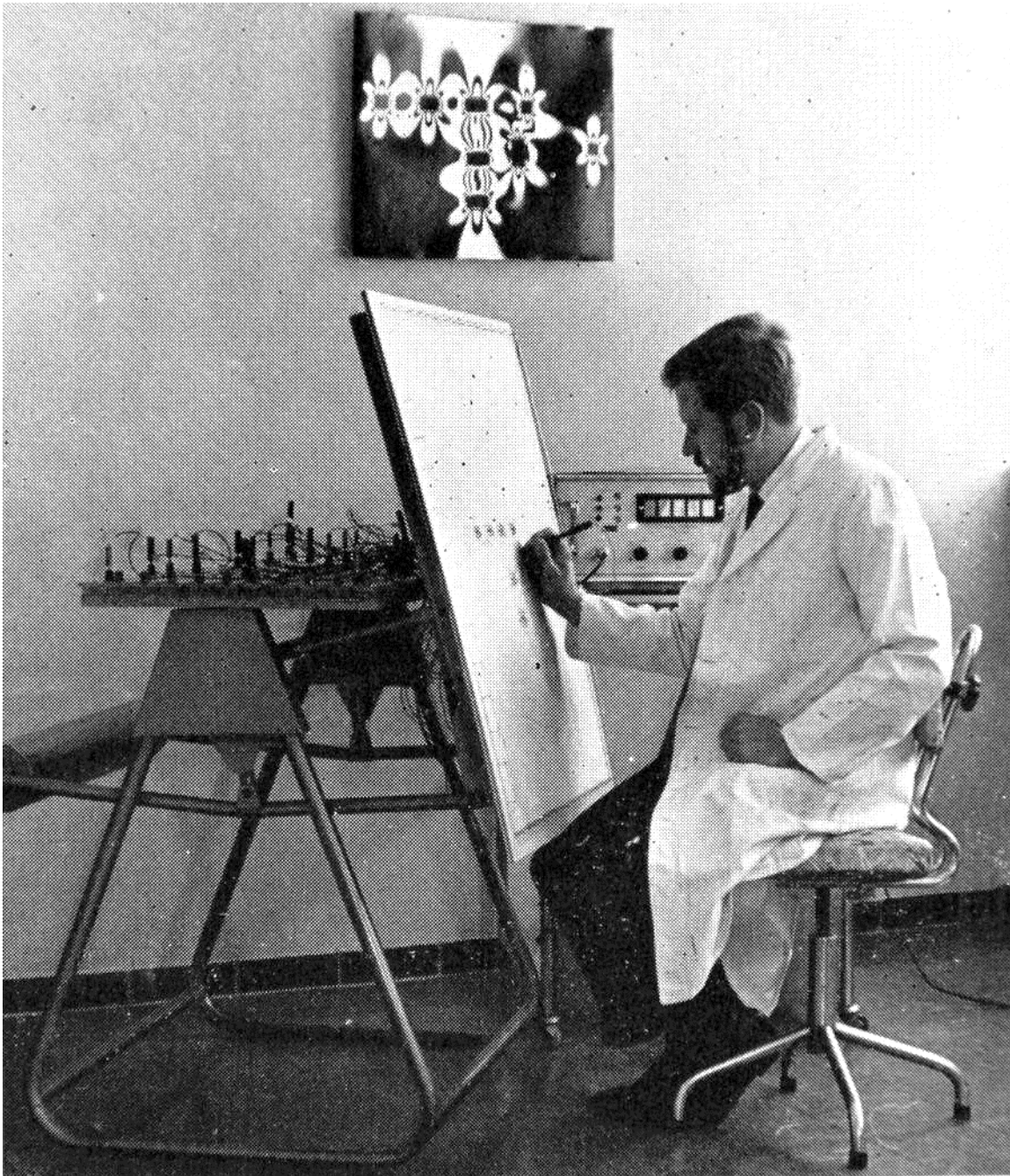
Figure 2. Conducting paper analogue for the solution of the La Place equation.
