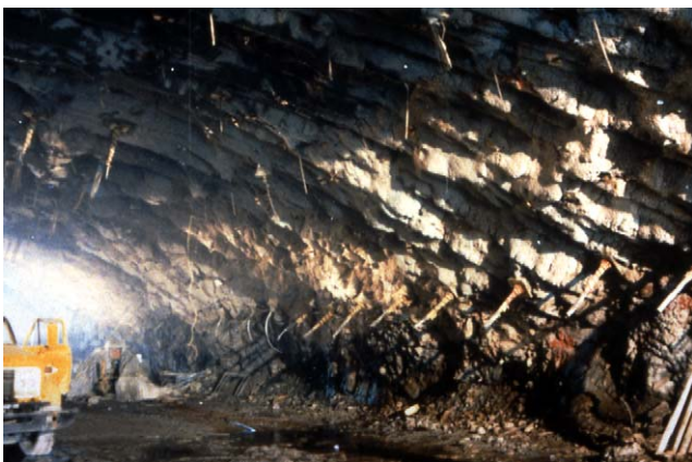
Fig. 17. Cavern profile achieved by drill and blast excavation in jointed sandstone.
