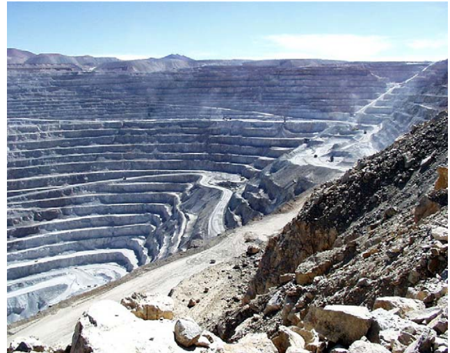
Fig. 15. Excavated slopes in the Chuquicamata open pit mine in Chile. These slopes are 850 m high and individual rock mass units are treated as homogeneous.
