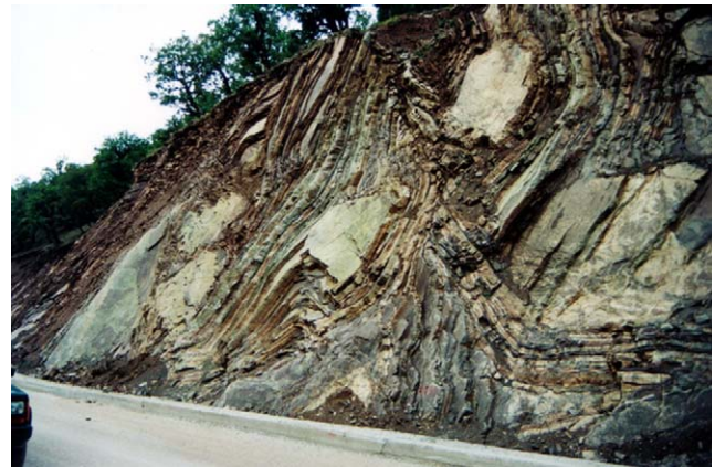
Fig. 19. Exposure of folded sedimentary rocks in a carefully excavated road cutting in the vicinity of the Acheloos tunnel in Greece.
