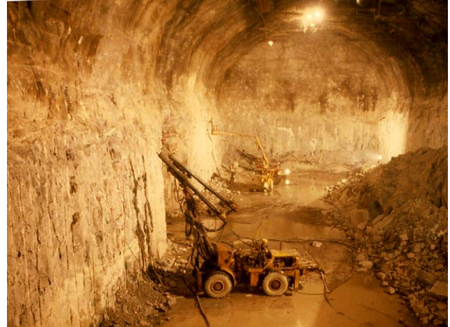
Fig. 18. Undisturbed conditions achieved by smooth blasting in massive gneiss in the underground powerhouse cavern of the Rio Grande Pumped Storage Project in Argentina.
