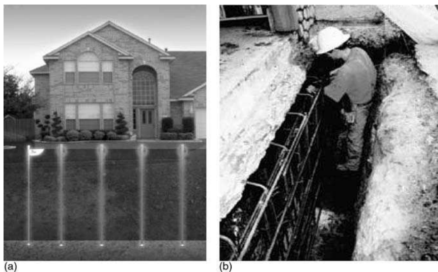
FIGURE 9.59 Illustration of underpinning. (a) Underpinning with mini-piles. (b) preparation of foundation for underpinning. (From www.saberpiering.com . With permission.)
