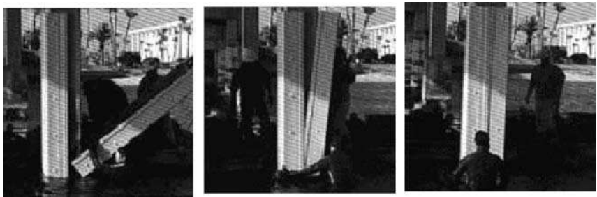
FIGURE 9.58 Replacement conventional pile jackets with lifejackets on Anna Maria Island Bridge. (Courtesy of Manatee County, Florida.)
