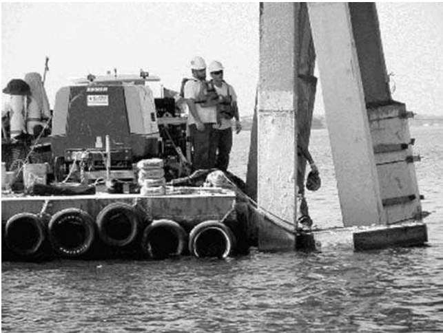
FIGURE 9.57 Installation sequence of pile jacket form. (Courtesy of Alltrista Co.)
