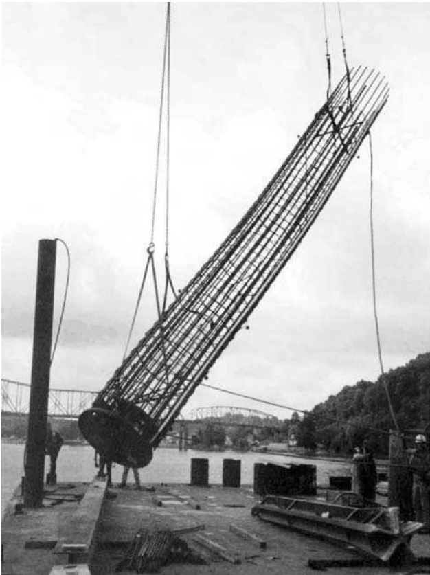
FIGURE 9.30 O-cell and cage lifted for installation. (Courtesy of LoadTest, Inc.)
