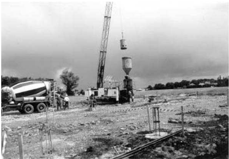
FIGURE 6.29 Filling of funnel and tube with concrete. (From Van Impe, W.F., 2004, Two Decades of Full Scale Research on Screw Piles . With permission.)
