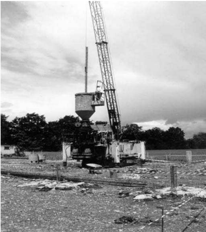
FIGURE 6.28 Installation of the reinforcement cage. (From Van Impe, W.F., 2004, Two Decades of Full Scale Research on Screw Piles . With permission.)
