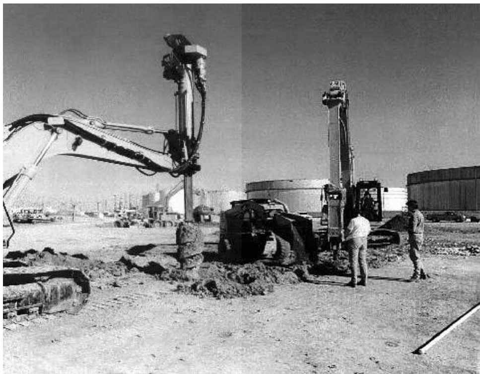
FIGURE 12.32 Installation of rammed aggregate piers, a type of stone column. (From Geopiers Foundation Co. With permission.).
