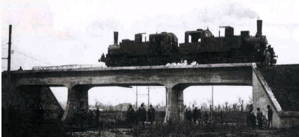
Bridge on Lorgana Canal on Bologna-Portomaggiore railway. Bridge testing.
