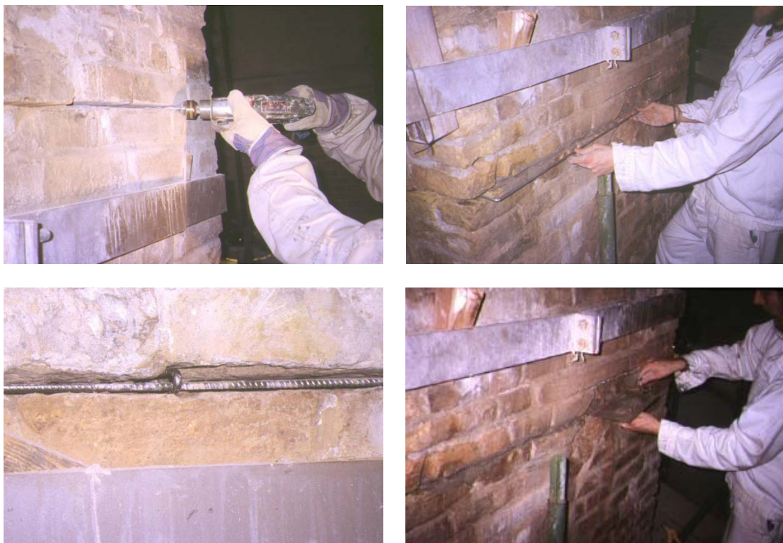
Figure 7: Steps for reinforced repointing intervention ([2] p. 443, fig. 3.24)
