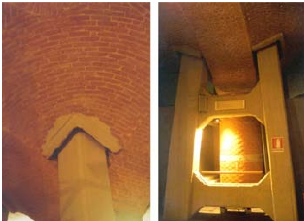
Figure 12: R.C. structure substituting the original one in the "Mole Antonelliana", Turin, Italy
