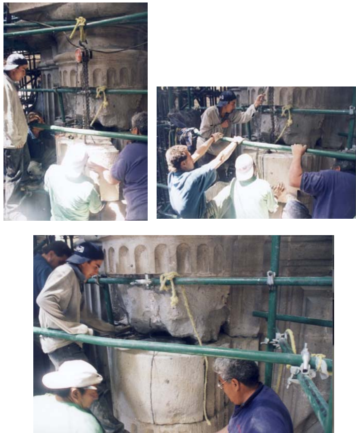
Figure 13: Substitution of individual blocks of a pillar in the Mexico City Cathedral [21]
