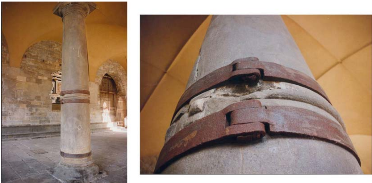
Figure 10: Local confinement for critical sections of a pier
