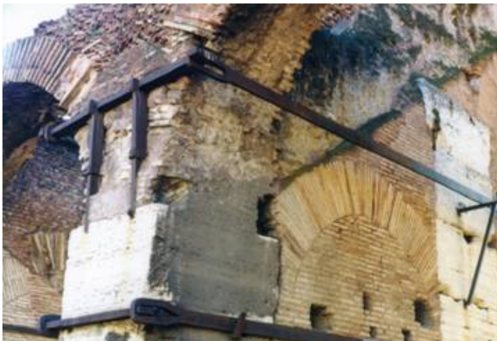
Figure 9: Example of anchoring with steel ties on a part of Coliseum, Rome, Italy
