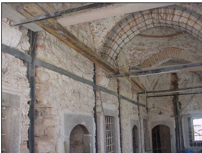
Figure 21: Steel frame structure substituting the load bearing wall
