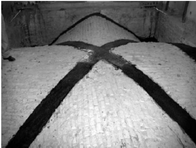
Figure 5: Strengthening intervention of cross vaults in the Town Hall of Assisi ([27] fig. 20)
