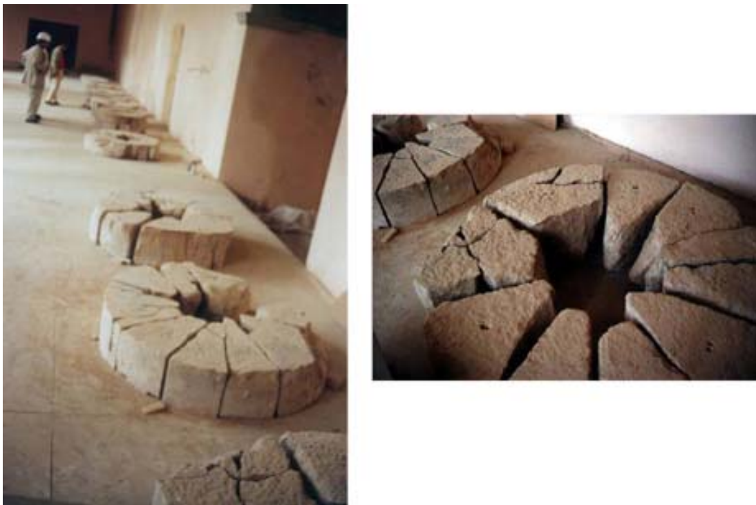
Figure 11: Removal of a pier of Tarazona Cathedral, Spain
