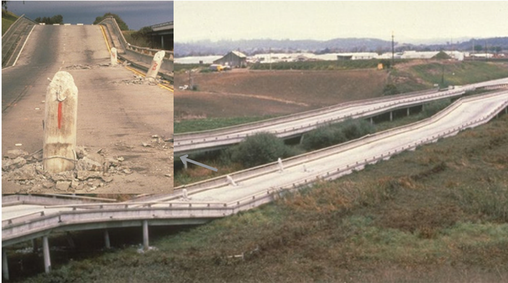
Figure B.43 Punching of piles through the road bed of the State Route 1, Watsonville area, span during the 1989 Loma Prieta earthquake. (After NISEE, 2000.)
