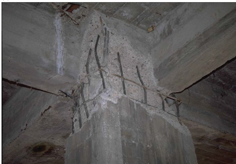
Inadequate number of stirrups at the beam-to-column connection
