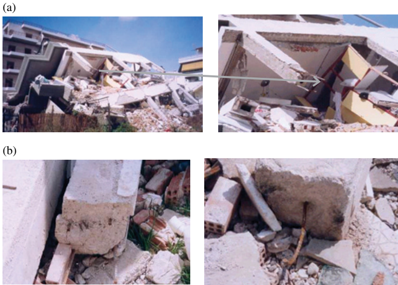
Figure B.19 Collapse of framed structure caused by inadequate anchorage of column longitudinal reinforcement bars in the 1999 North Athens earthquake: collapsed frames (a) and close-up of the pull-out of the steel bars (b).
