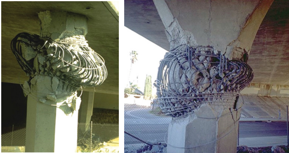
Figure B.46 Confinement failure at a bridge pier top during the 1994 Northridge earthquake. (After NISEE, 2000.)
