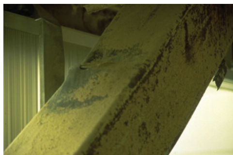
Figure B.31 Typical local (a) and global (b) buckling of diagonal braces. (After NISEE, 2000.)
