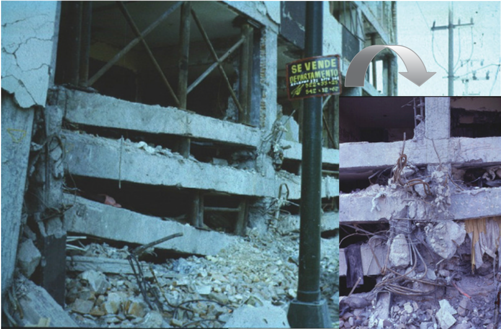
Figure B.13 Soft storeys in multi-storey RC frame caused by resonance in the 1985 Michoacan (Mexico City) earthquake: collapsed frames and inset with close-up of the crushed columns. (Courtesy of Fischinger.)
