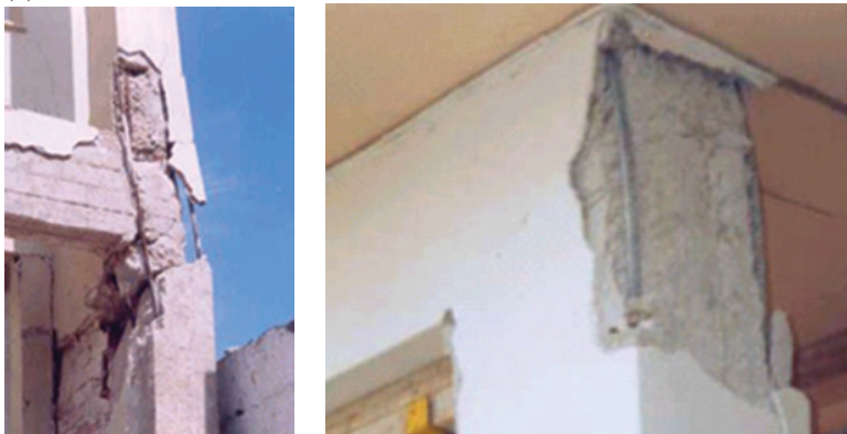
Lack of stirrups at the beam-to-column connection
