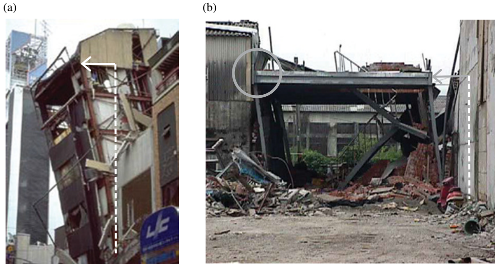
Figure B.37 Excessive lateral displacement during the 1995 Kobe, Japan, (a) and the 1999 Chi-Chi, Taiwan, earthquake (b). (After FEMA 355E, 2000.)
