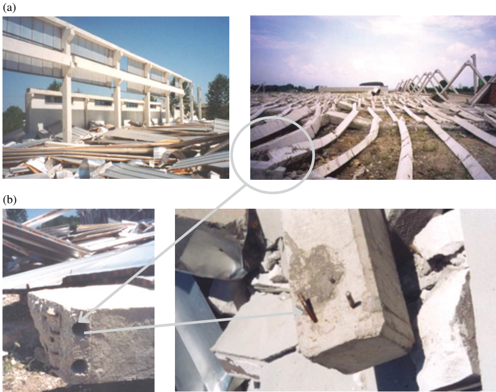
Figure B.16 Collapse of precast RC building during the 1999 Kocaeli earthquake: general damage (a) and close-up of the details (b).
