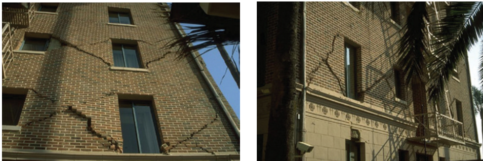
Figure B.11 Diagonal cracks in the infills of an apartment building on Wilshire (Santa Monica, California) in the 1994 Northridge earthquake. (After NISEE, 2000.)
