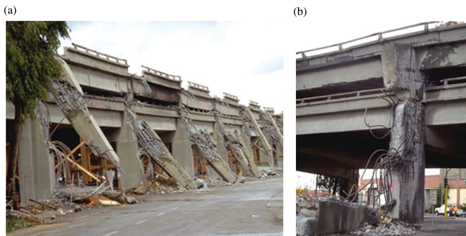
Figure B.55 Sliding shear at top columns of the Cypress viaduct in the 1989 Loma Prieta earthquake. (After NISEE, 2000.)
