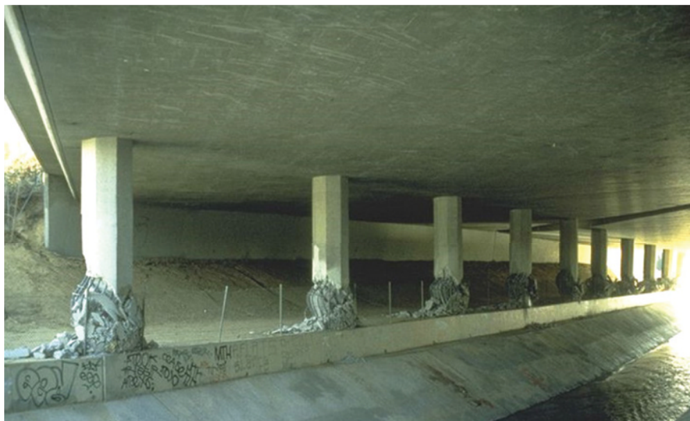
Figure B.47 Flexural plastic hinges in columns connected by a wall, Bull Creek Canyon Channel bridge, 1994 Northridge earthquake. (After NISEE, 2000.)
