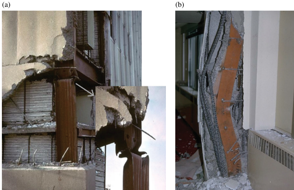
Figure B.29 Buckling in columns of the Cordova Building during the 1964 Alaska earthquake: local buckling (a) and member buckling (b). (After NISEE, 2000.)
