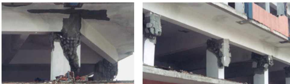
Figure B.4 Shear failures in short columns observed in the 1999 Kocaeli (Turkey) earthquake.
