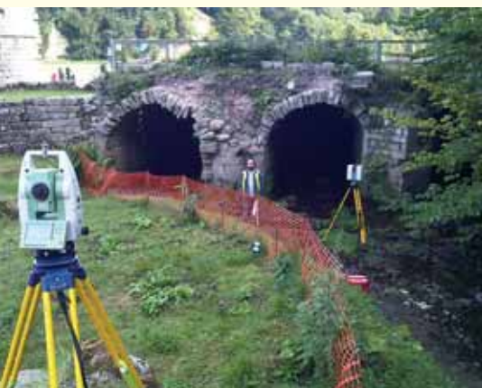
Fig CS4.1 Surveying the tunnel entrances.
