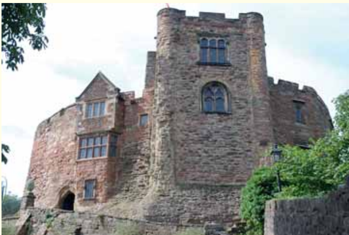
Fig CS9.1 Tamworth Castle; the shell keep looking from the causeway used to approach the castle.
