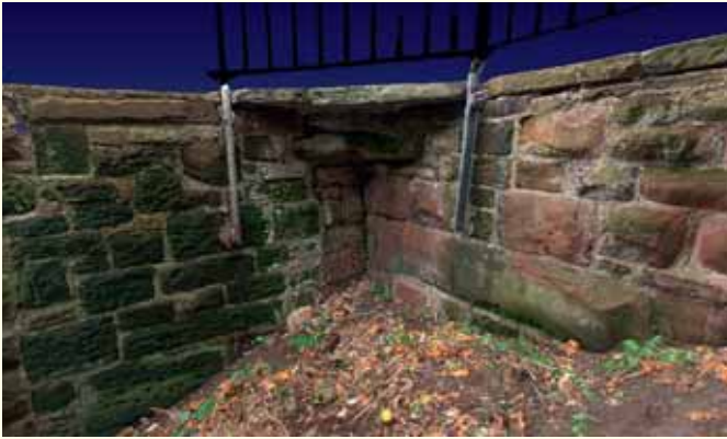
Fig CS12.2 Colourised point cloud data after digital removal of vegetation in foreground.
