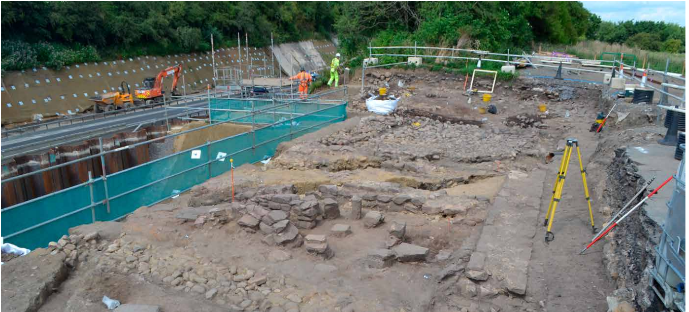
Figure CS1.2 A general view of the excavations taking place at Fort Bridge.
