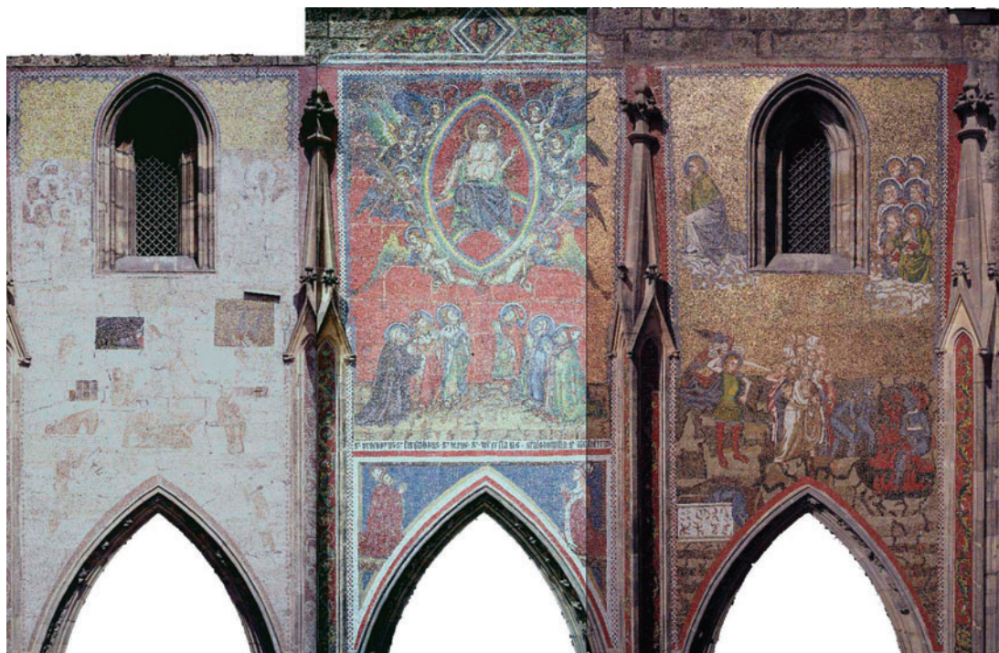
Rectified images of the facade, showing its state before conservation ( left ), after treatment ( center ), and after gilding ( right ). Images: Jaroslav Zastoupil.
