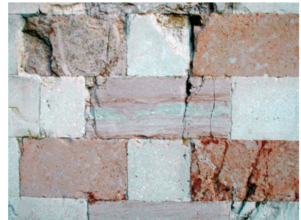
Detail showing the masonry deterioration of the facade caused by seismic stress. Photo: © Marco Tallini.
