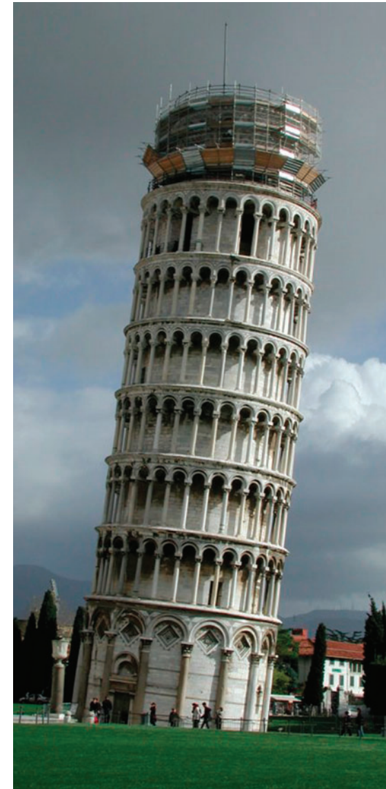
The Tower of Pisa in 1993, with its belfry under conservation during the preliminary stabilization phase. Photo: © Gary Feuerstein, 1993.
