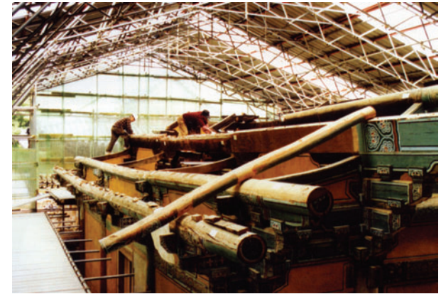
The Hall of Paradise, during restoration. Dismantlement of the temple allowed each building component to be documented individually. Photo: © Soon-Kwan Kim.
