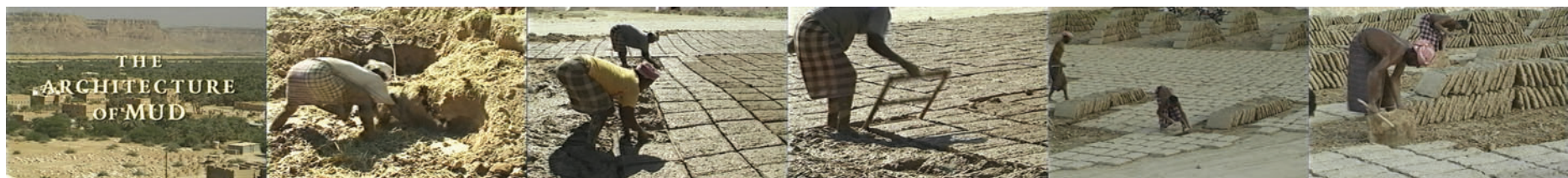
Series of stills from the documentary, showing workers in Seyoun creating mud bricks for new construction. Soil is gathered and mixed with straw and water. The mixture is spread out evenly in a mold, which is lifted immediately. The mud bricks are then left to dry in the sun for a week. Photos: © Caterina Borelli.
