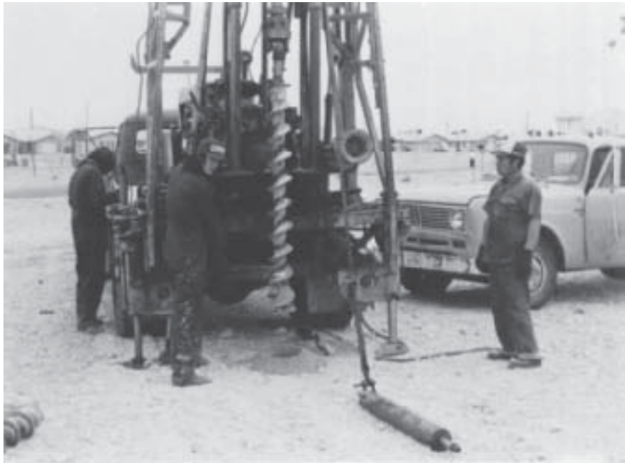
Figure 10.3 Drilling with continuous-flight augers (Courtesy of Danny R. Anderson, Danny R. Anderson Consultants, El Paso, Texas)
