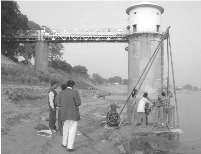
FIGURE 10.3 Wash boring method.
