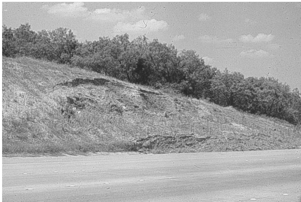
FIGURE 8.10 Typical slope failure in expansive clay.
