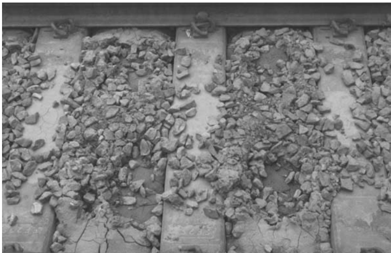
FIGURE 14.12 Migration of fines from subgrade into ballast.
