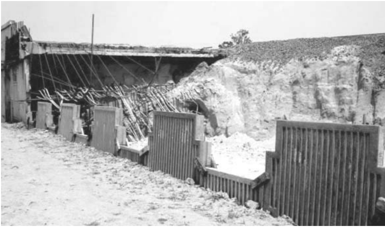
FIGURE 6.29 Failure of mechanically stabilized retaining wall due to rupture of ties.
