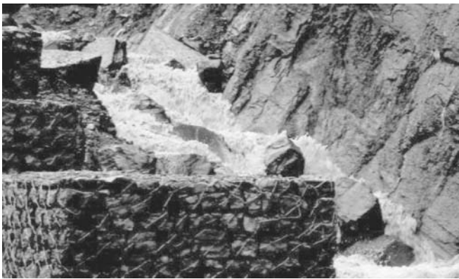
FIGURE 6.4 Gabion wall.
