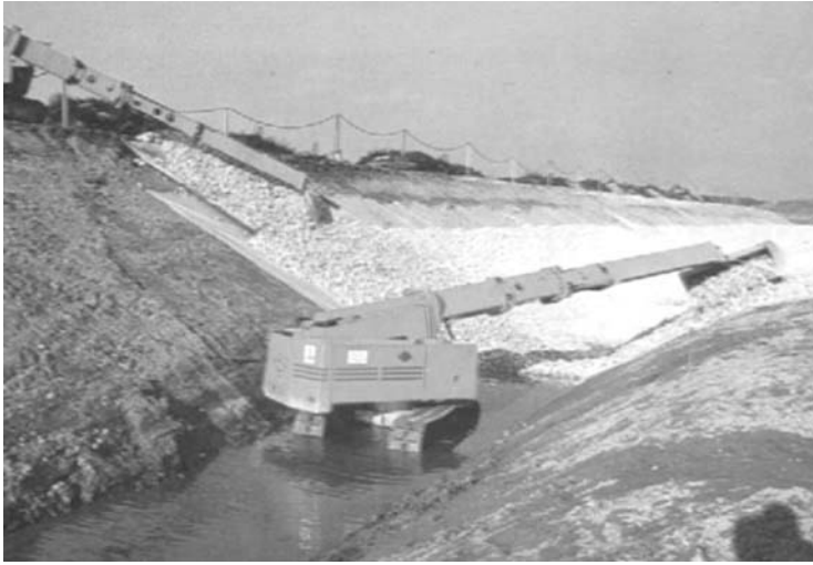
FIGURE 12.8 Geotextile filters in stream bank protection.
