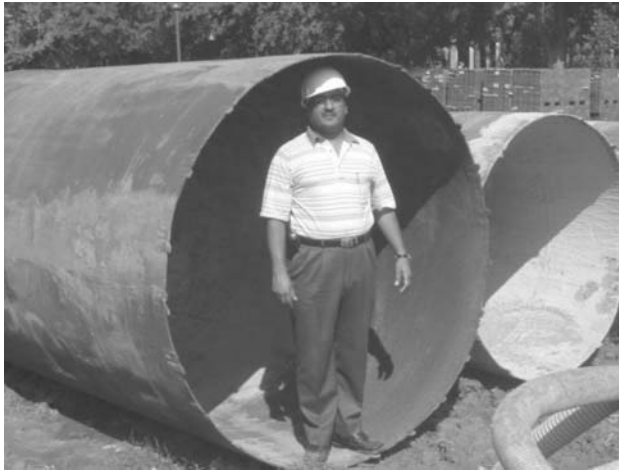
FIGURE 5.7 Steel casing for construction of drilled shafts.
