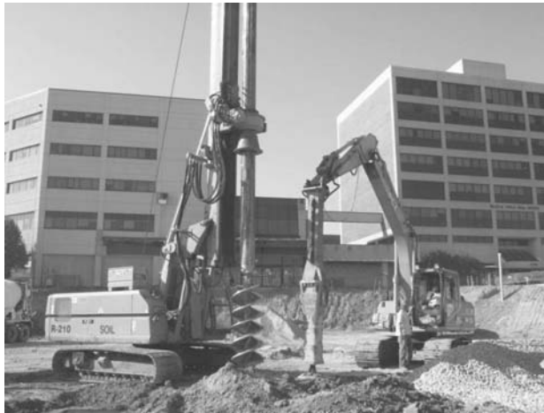
FIGURE 5.8 Construction of a geopier.
