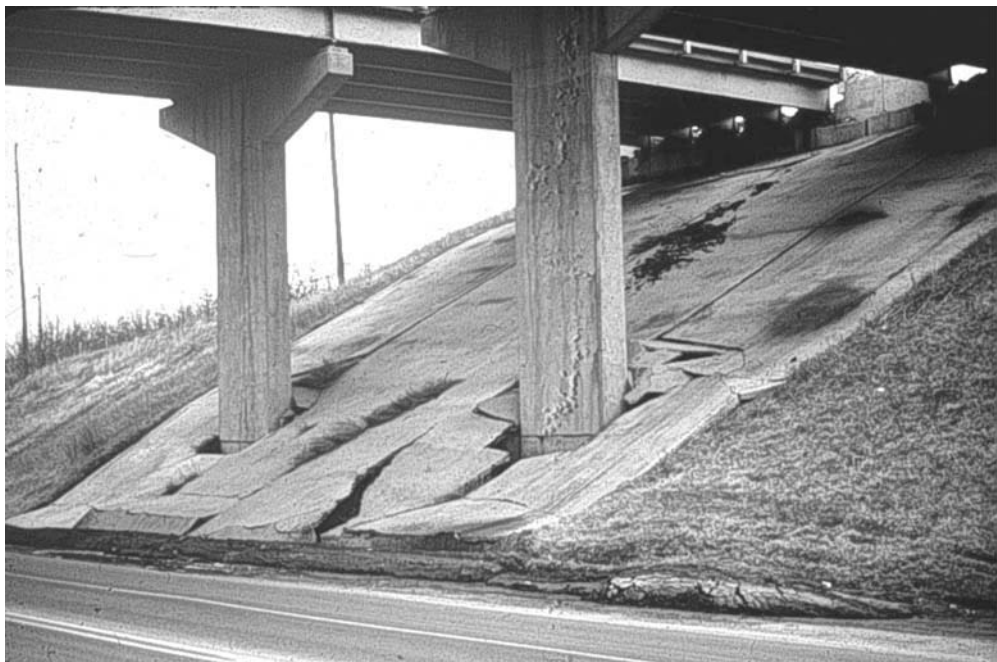
FIGURE 8.9 Slope movement under bridge and against supports.
