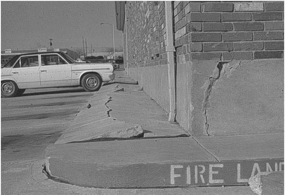
FIGURE 8.1 Typical distress caused by expansive clays.
