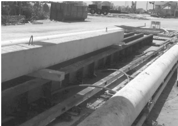
FIGURE 5.6 Reinforced concrete square and circular piles.
