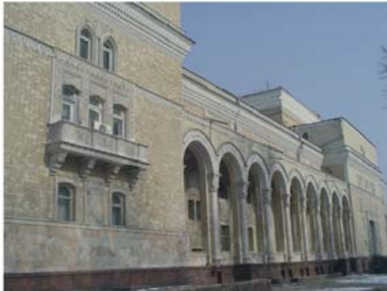
FIG. 15(a-b). Tashkent. Alishir Navoi Theatre. 1936–47. Architect: A. Shchusev. (Photos: Courtesy of M. Azzout and G. Akramova.)
