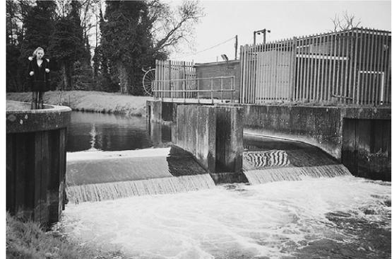
**Fig. 6.28** Marham gauging station on the River Nar, Norfolk, England (NGR TF 723 119; catchment area 153.3 km<sup>2</sup>; mean flow 1.15 m<sup>3</sup> s<sup>-1</sup>). The gauging structure is a critical depth flume, 7.16 m wide. The stilling well is positioned behind the metal fence on the downstream, left wall of the flume. Prior to April 1982, the flume (7.47 m wide) contained a low flow notch at the centre. Weed growth can be a problem during summer if not cut regularly.
